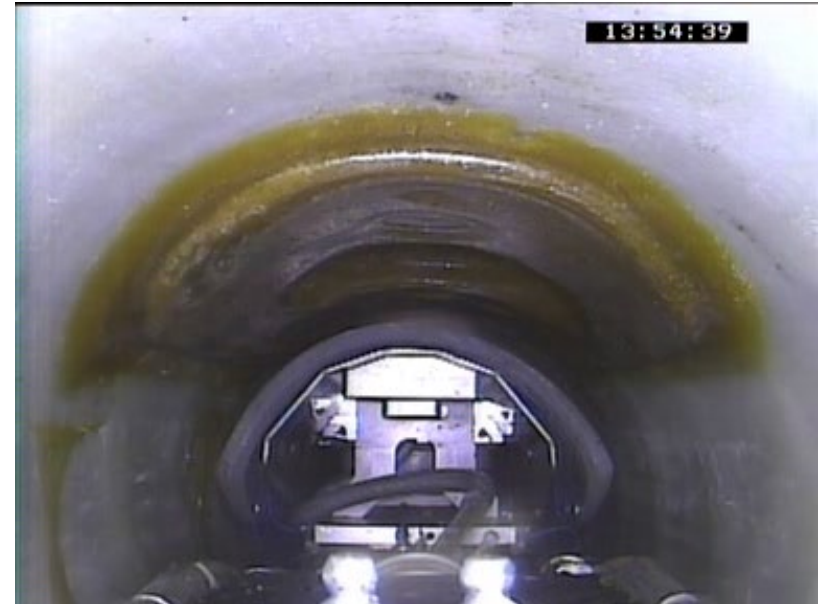
Repaired connection following repair using 2K Injection system
