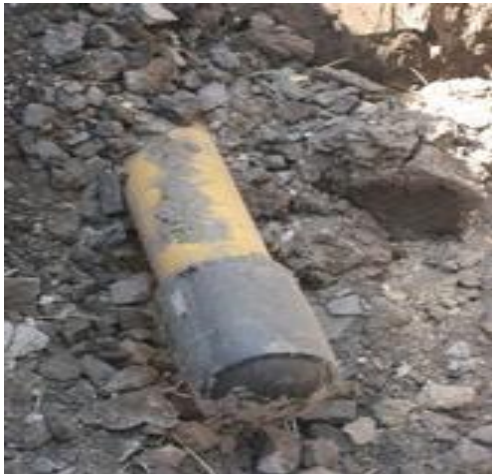
Sandless installation using the backfill creates point loads by stones
