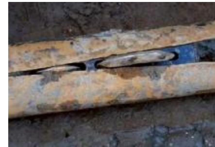
Cut Ductile pipes: ductile iron, lead, plastic
